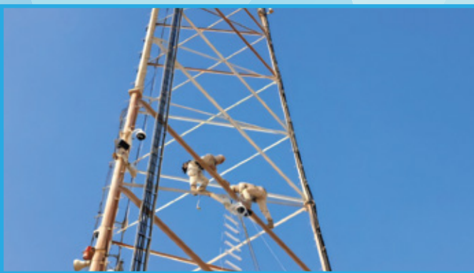
Signal Tower Maintenance (OKP-10, Sigs)
