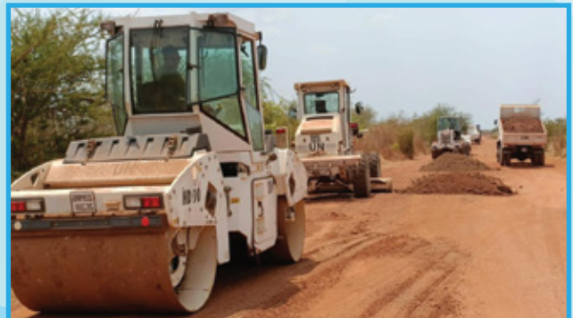
MSR Rehabilitation Project Work (BANENGR (RPF) COY-8, UNMISS)
