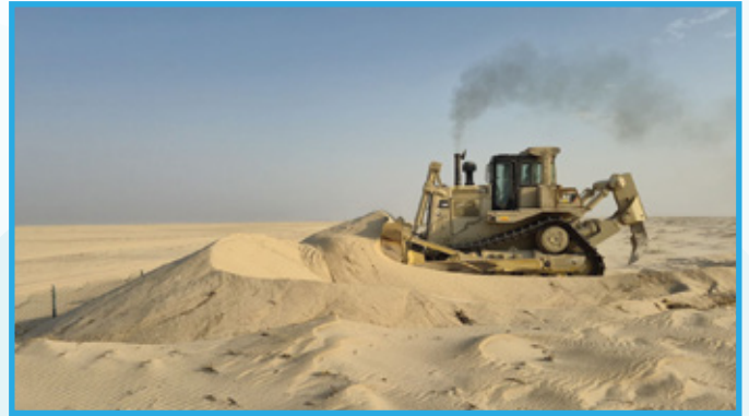
Construction of Sand Dam (OKP-8, Engrs)
